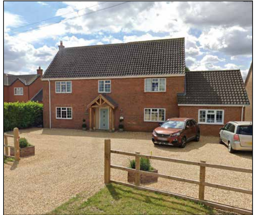
F.57: New house a mix of brick, tiles and wood. (Photo © Google Earth 2022)
