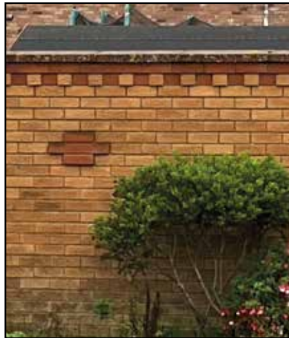
F.31: White brick with red brick detailing. (Photo © AECOM 2022)
