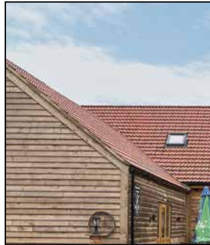
F.32: Wood cladding. (Photo © AECOM 2022)
