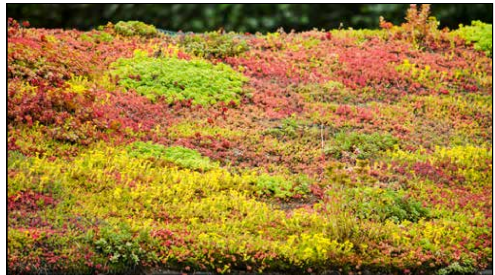
Figure 75: Natural flood prevention, green roof as part of a SuDS management system.
