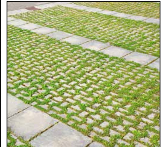
Figure 71: Permeable paving. (Photo © Adobe Stock 2022)
