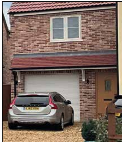
F.27: Casement window mirroring traditional sash style and covered porch. (Photo © AECOM 2022)
