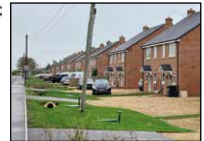
Figure 61: New builds with open swales marking the boundary. (Photo © AECOM 2022)
