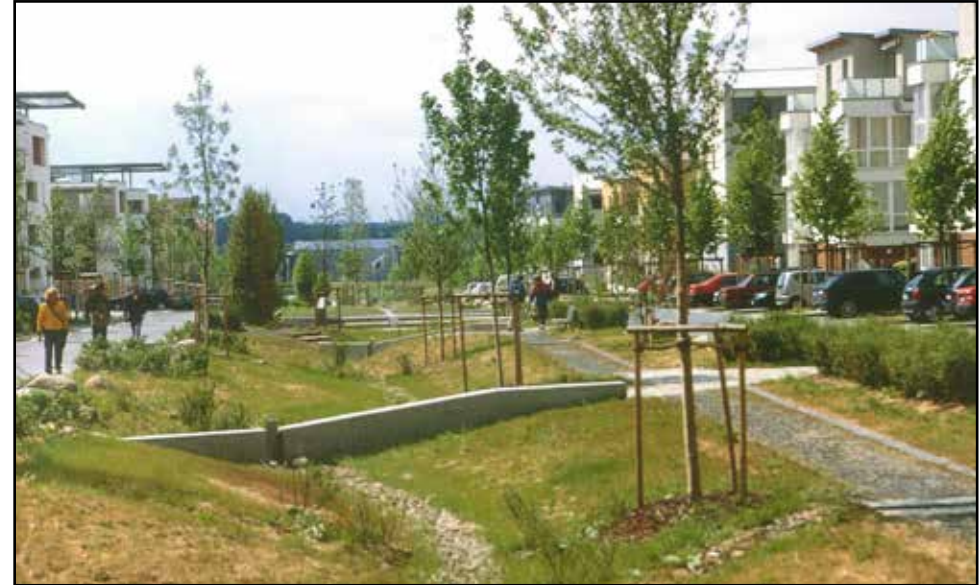
Figure 74: Natural flood prevention, swale as part of a permeable landscape.
