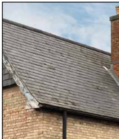
F.35: Slate roof. (Photo © AECOM 2022)
